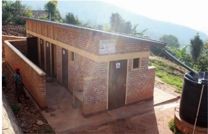
The new latrine constructed at Ngoma School in Rwanda includes 12 stalls. Photo credit: WFP
